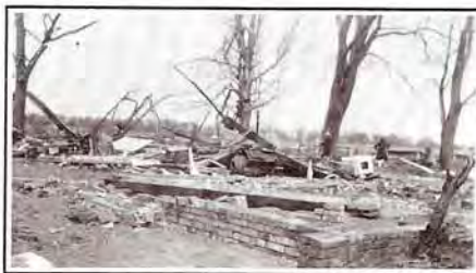
Oakland School site after the 1927 tornado. Courtesy of Dorothy Kline.
